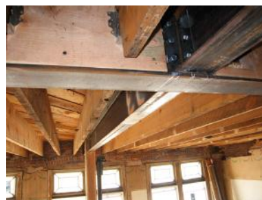
Close up view of the steel beams
