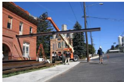
Placing steel inside the building
