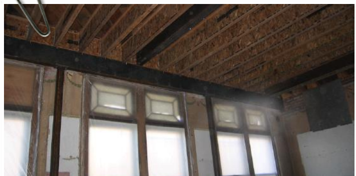
Dinning room steel beams and posts
