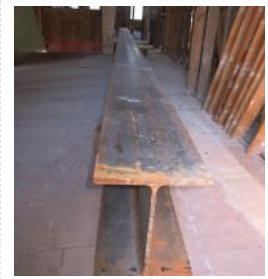
Steel beam upstairs
